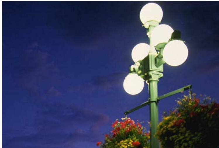
Streetlights with five fixture heads per pole
