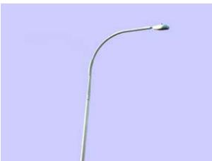
**Tully, Onondaga County** — To save energy, reduce light pollution and light trespass, the town of Tully retrofitted 24 lighting fixtures along Route 80. The previous fixtures, cobraheads containing 175 watt mercury vapor lamps, were replaced with flat-lens fixtures containing 100 watt high pressure sodium lamps. The primary purpose of the lighting in this installation is to aid driver and pedestrian visibility. **Contact: William Lund, Town of Tully, (315) 696-4693**
