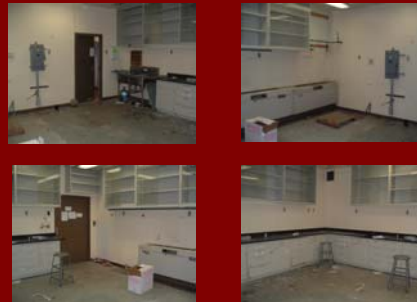
Process Room in Blaw Knox before renovation
